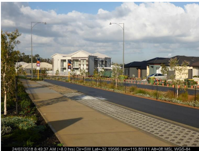
Photo ID: Photo 3 The infrastructure and housing west of the development site.
