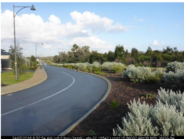
24/07/2018 8:52:54 AM (+8.0 hrs) Dir=W Lat=-32.19542 Lon=115.86092 Alt=3ft MSL WGS-84 Photo ID: Photo 10 Looking at the revegetated shrubs which on maturity will be less than 2 metres high.
